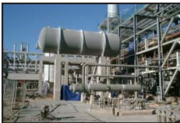
The new Axens unit under construction (Courtesy of Fluor Daniel)
